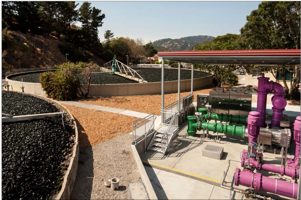
Trickling filters
