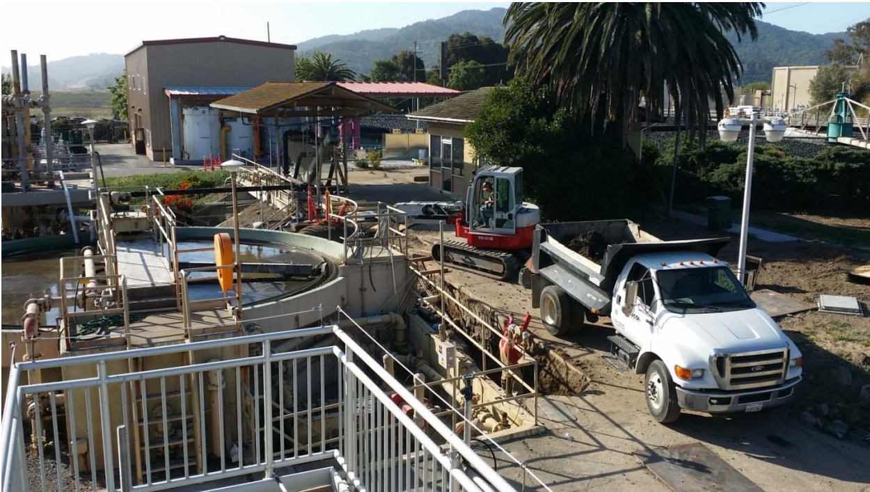
2015 Plant Improvement Project in Process
