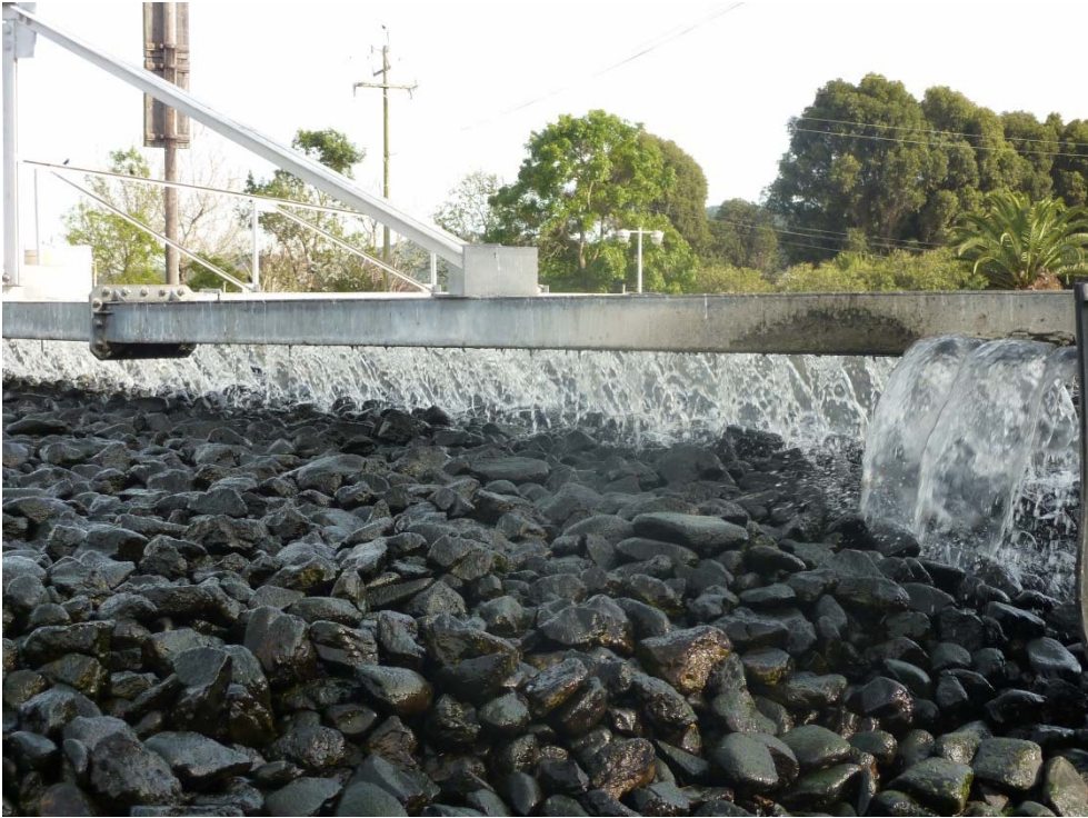
Trickling filters
