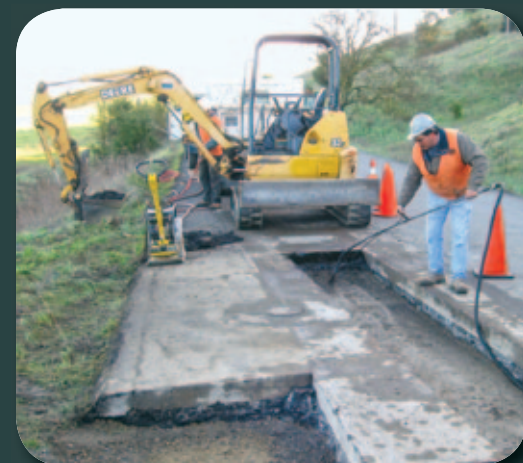
Installing corrosion protection on existing pipelines.
