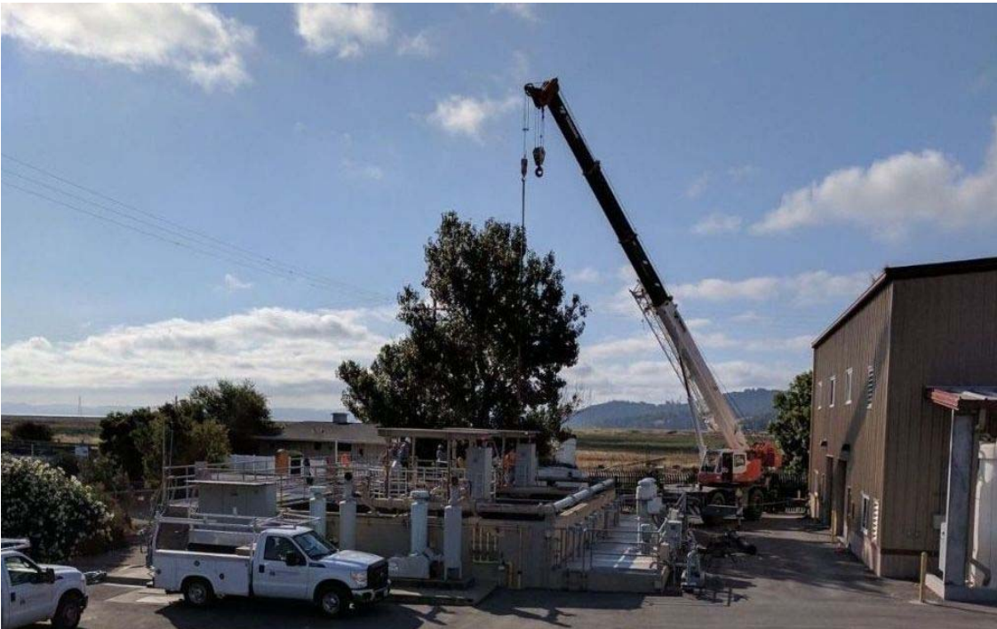
Deep Bed Filter Inlet Valve Replacement Project
