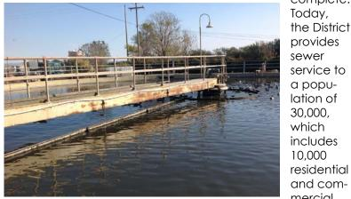
The Secondary Clarifier is used to remove floating solids and solids that have settled to the bottom. It no longer meets safety standards.
