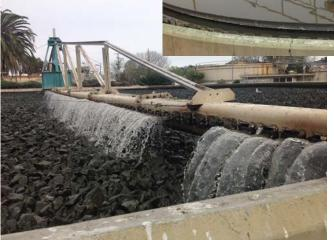
The trickling filters are part of the biological treatment systems. There is insufficient treatment capacity and it is unable to meet new requirements.
