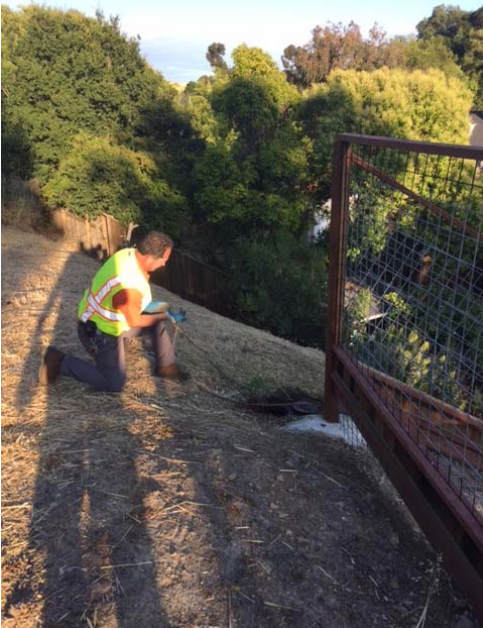
Inspecting a Sewer Easement
