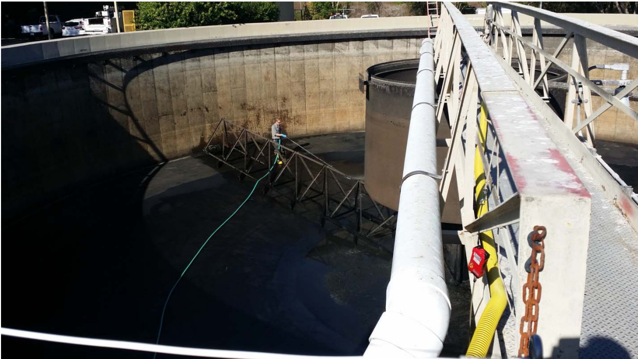
Primary Clarifier Drain, Clean, Inspect and Repair
