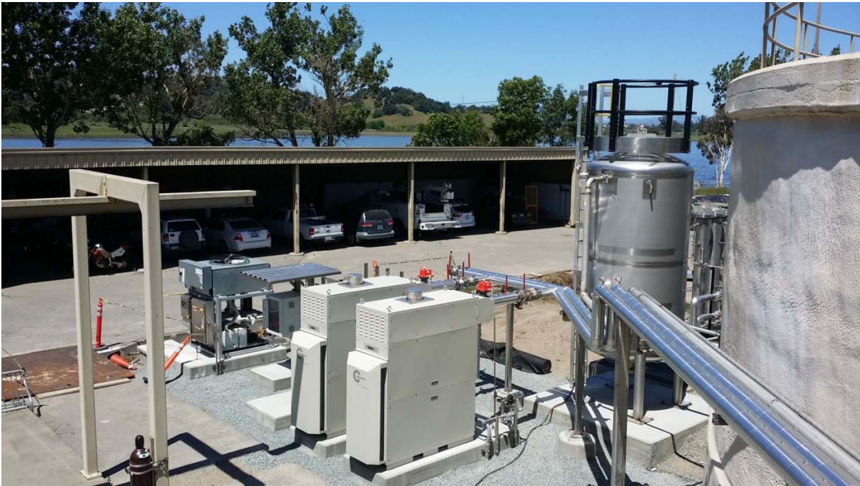
BERS Project Ready for May 9, 2016 Start Up
