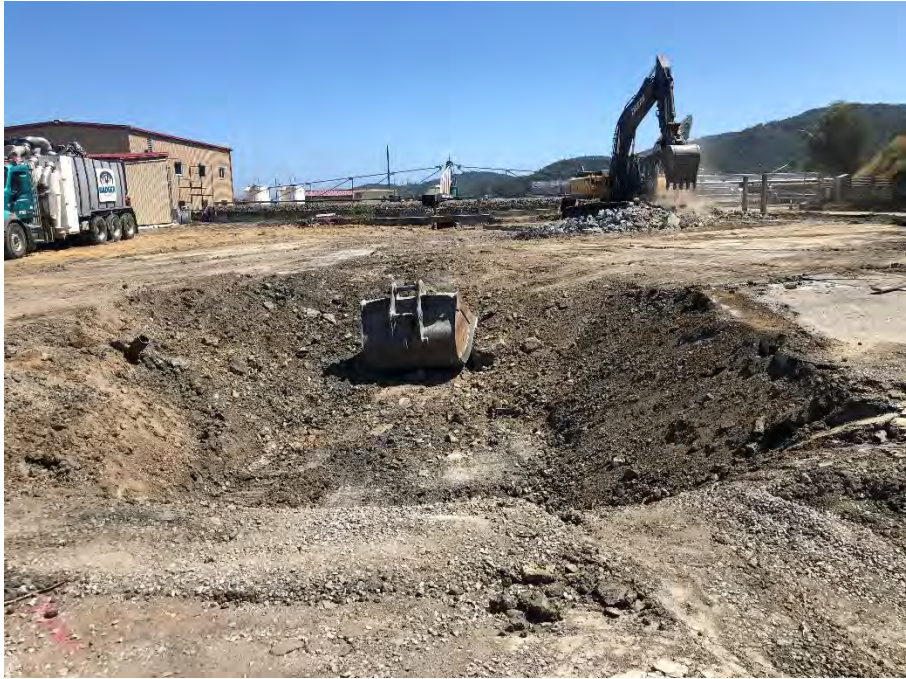
Demolition related to Treatment Plant Upgrade Project
