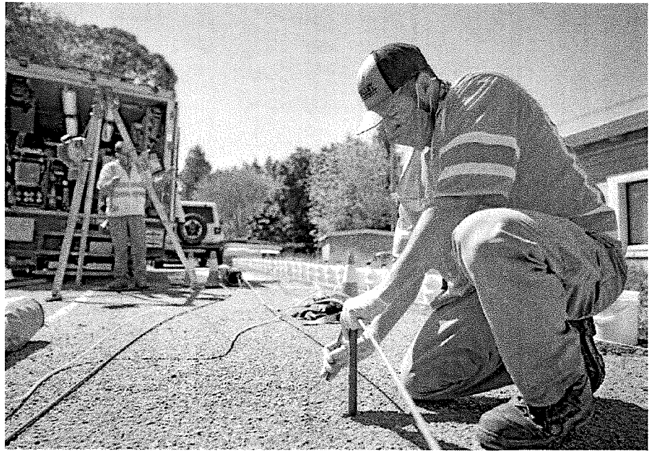
Ross Valley Sanitary District collections worker Ricky Smith prepares the inflation line for an epoxy patch carrier. Ross Valley is one of California's oldest wastewater utilities, with aging clay pipes that require regular maintenance and repair.
