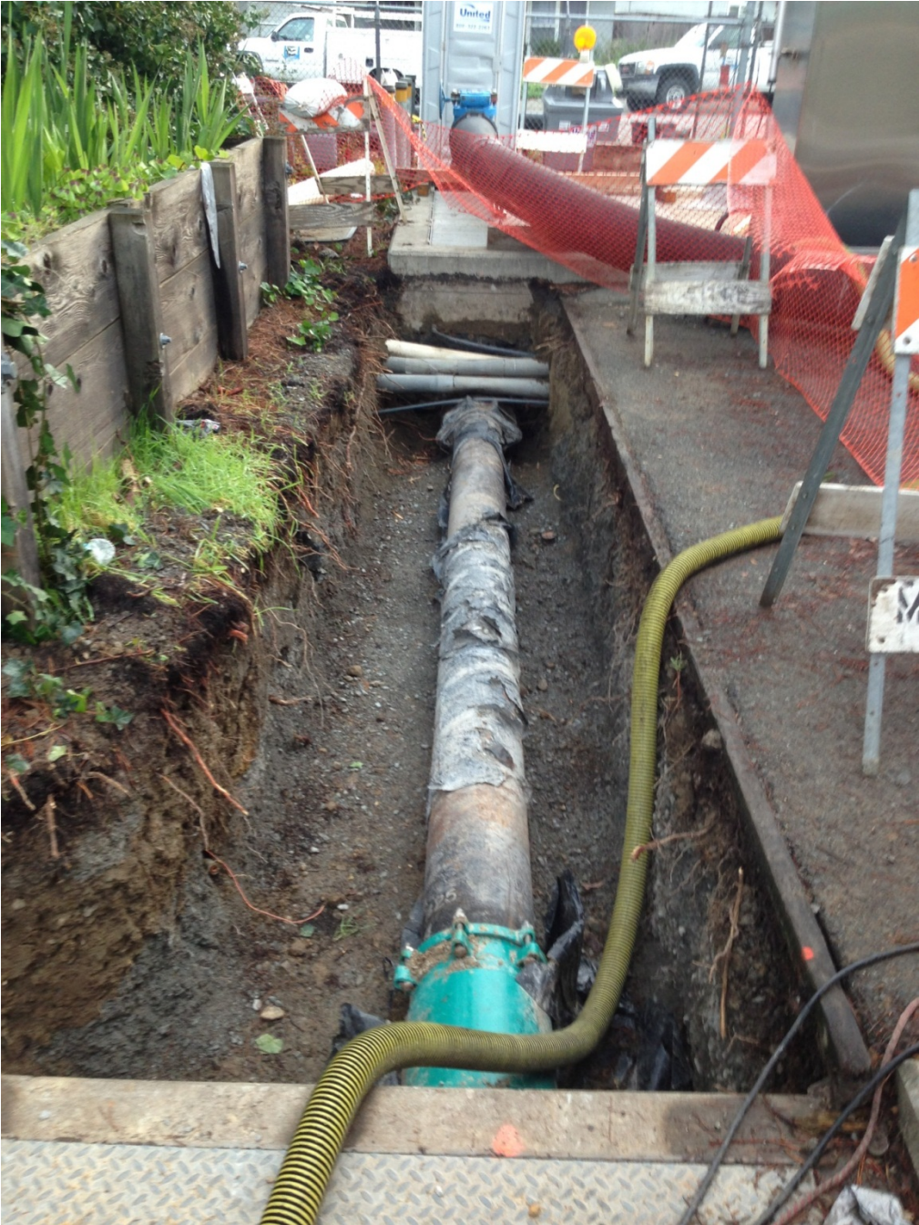
Descanso pump station construction
