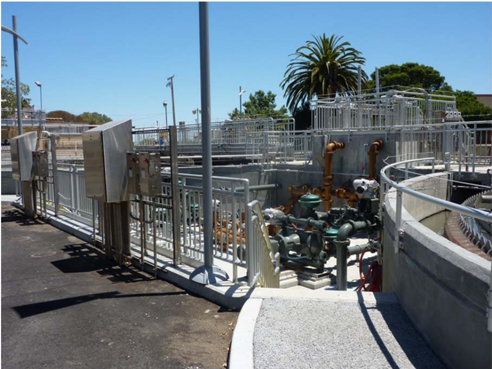
Treatment plant facilities
