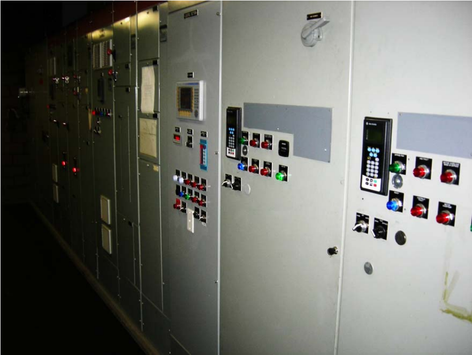
Treatment plant facilities
