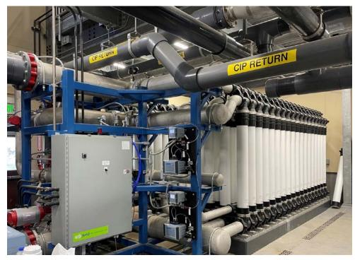
Recycled water membrane filter system
