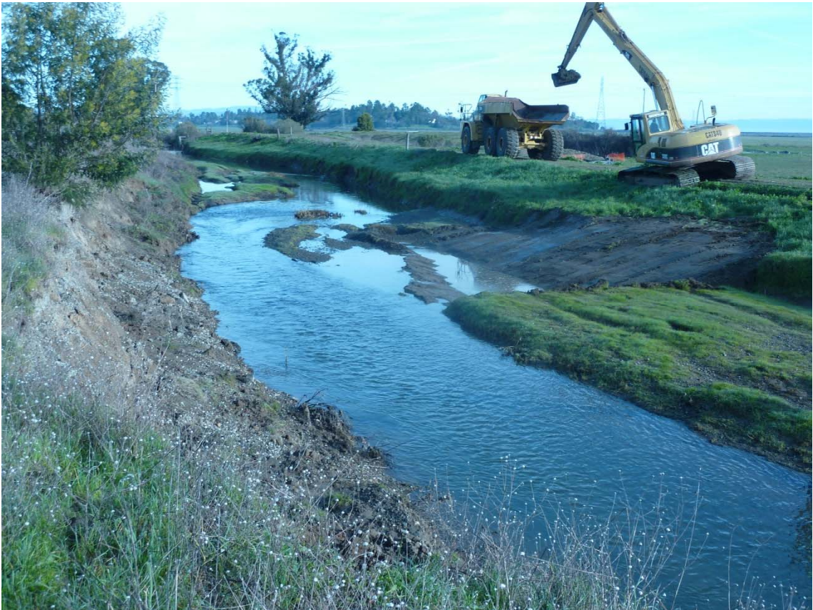
Emergency Miller Creek levee repairs due to rain
