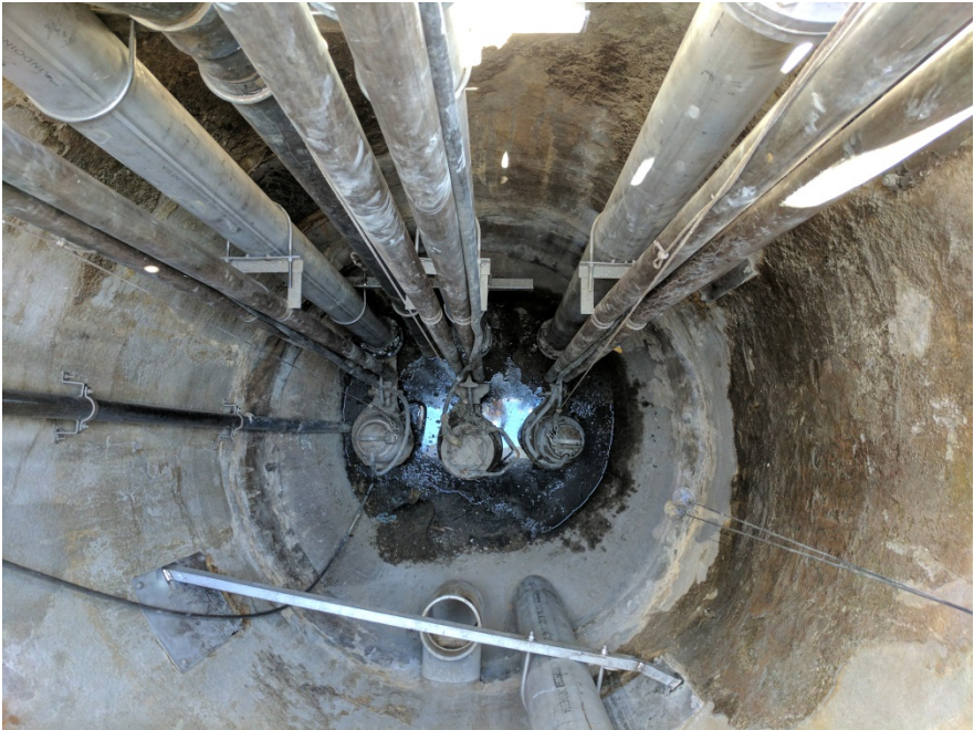
Descanso pump station wet well upgrade project
