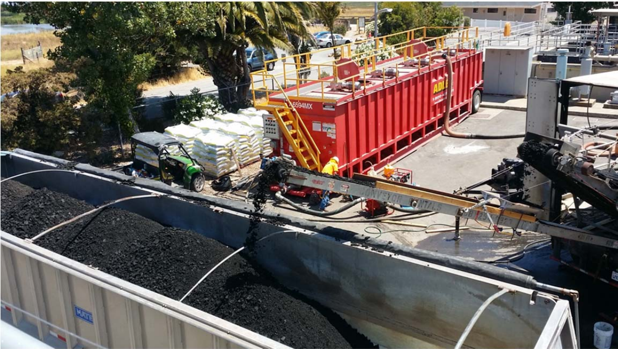
Primary digester cleaning project sludge dewatering process
