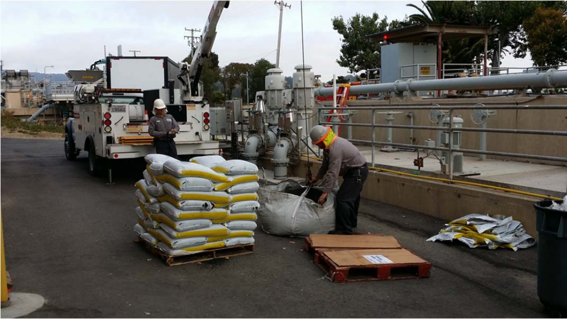
Employees performing maintenance work at the District
