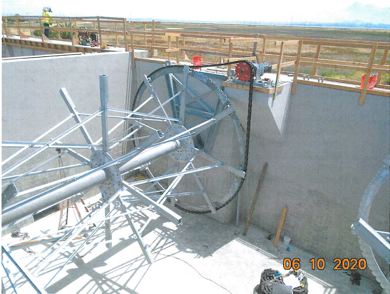
Figure 1. Construction of Bio-Wheels. Photo taken on 6/10/2020.
