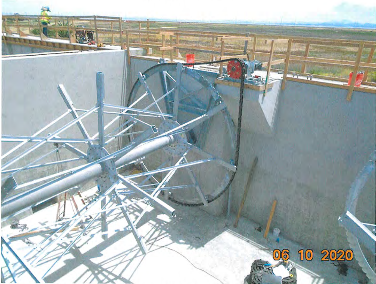
Figure 1. Construction of Bio-Wheels. Photo taken on 6/10/2020.
