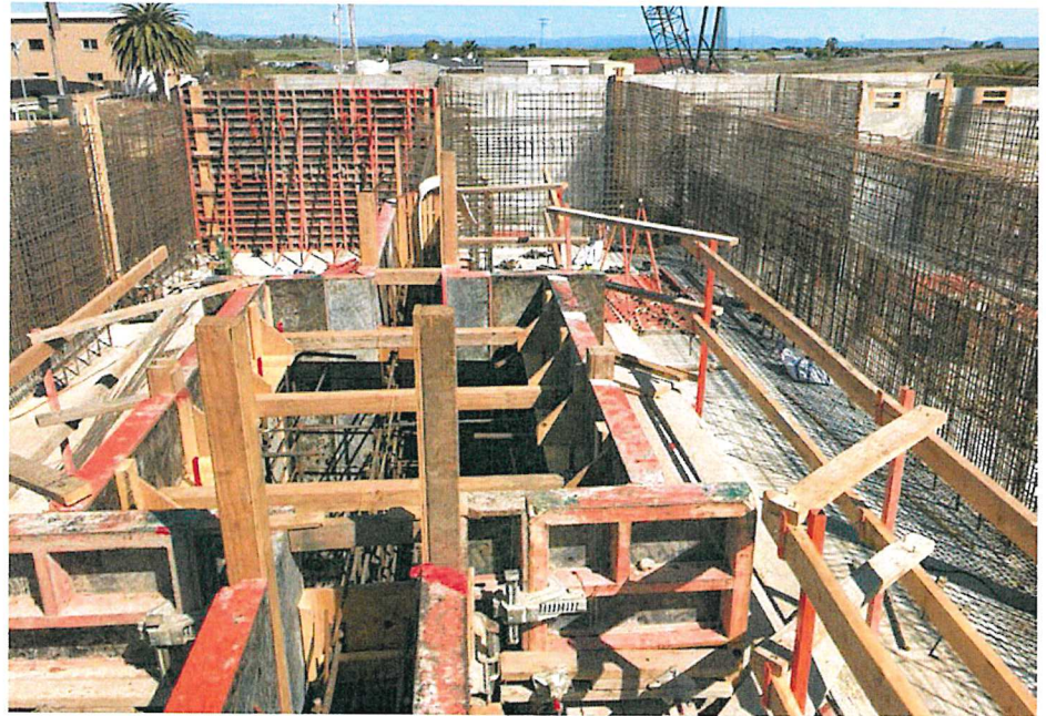
Aeration basin interior walls formwork and rebar.
