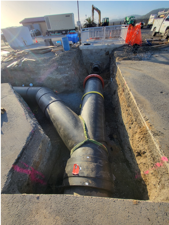
Secondary Effluent Line Modifications Project
