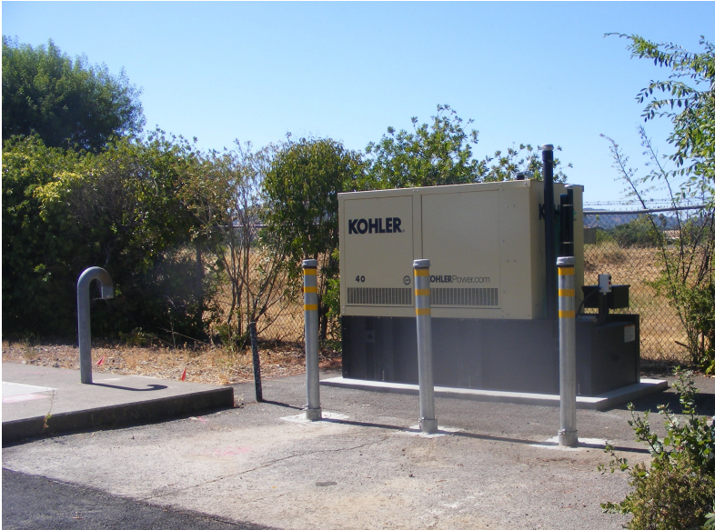
Standby Generator System Installation at Pump Station
