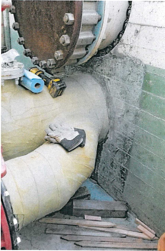
Figure 1. Manifold – Before Construction
