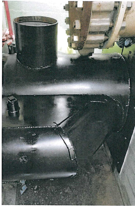
Figure 2. Manifold – After Construction
