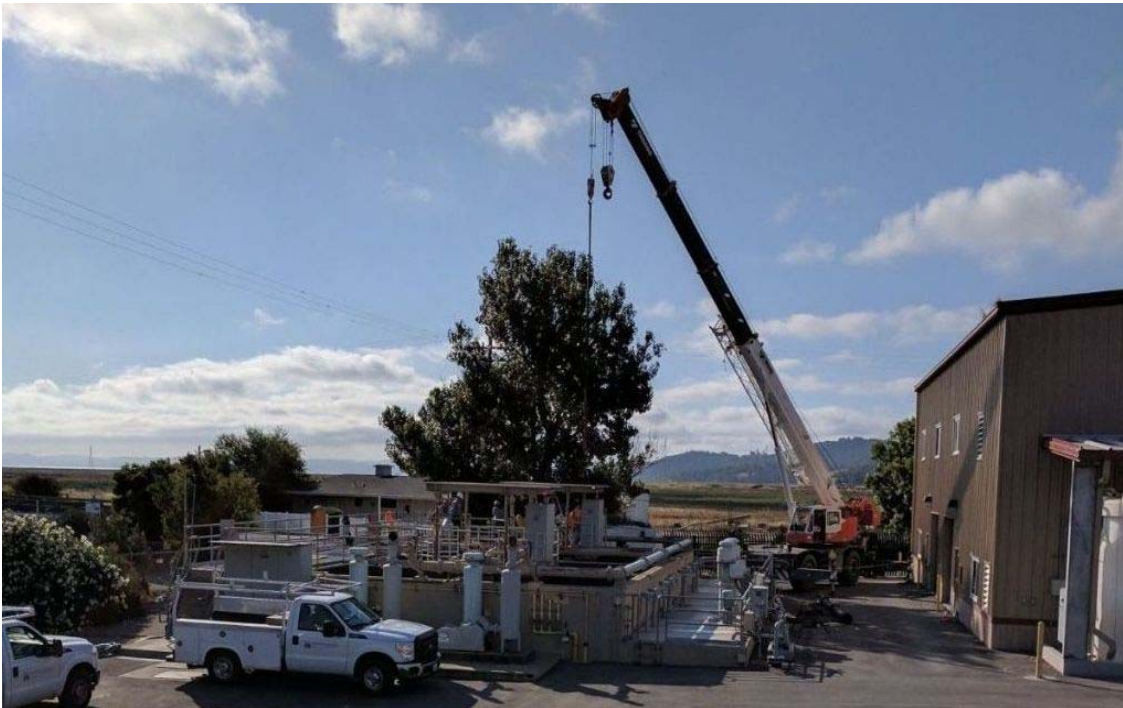
Deep Bed Filter Inlet Valve Replacement Project
