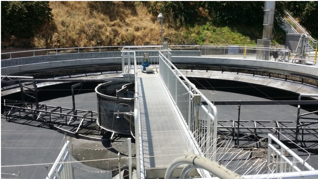
Primary Clarifier #3 drained, inspected and Stamford baffles removed
