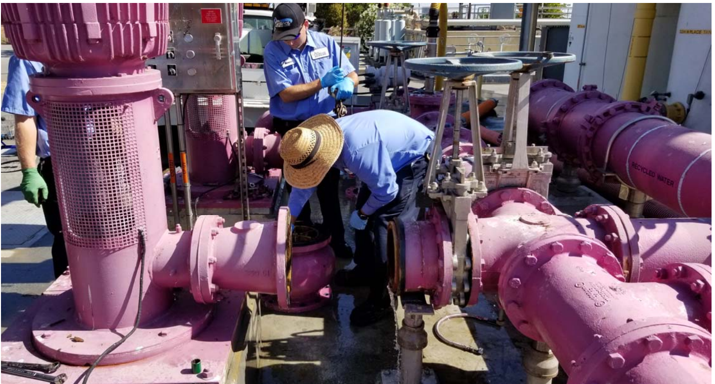
Staff Repairing NMWD Distribution Pump Check Valve
