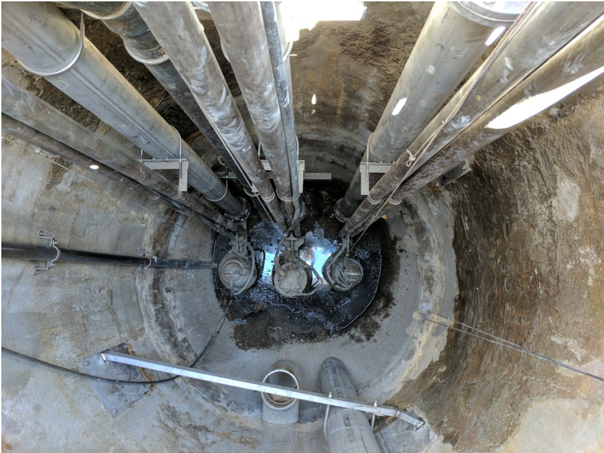
Descanso pump station wet well upgrade project
