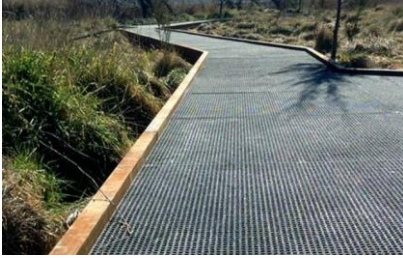
4 Elevated ramps & deck
