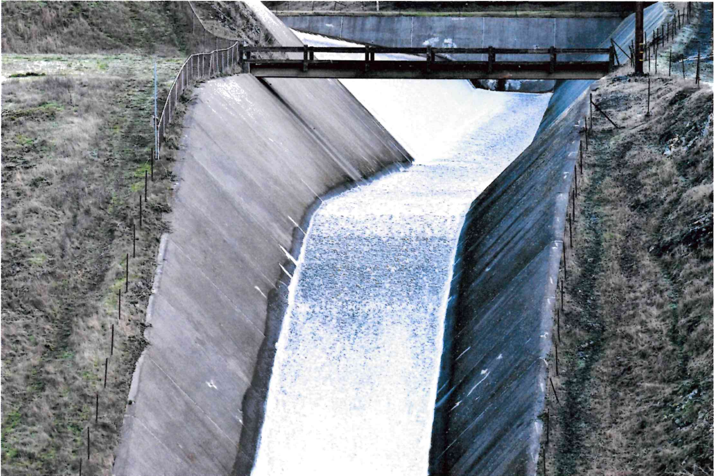
Water flows over the spillway at the Nicasio Reservoir. The Nicasio project would modify the reservoir's spillway gates to add 3,000 acre-feet of water storage. ALAN DEP – MARIN INDEPENDENT JOURNAL, FILE
