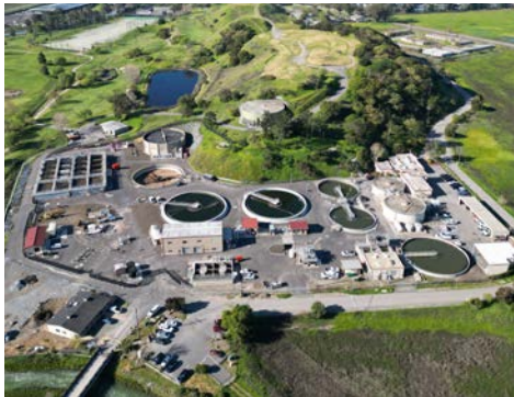
District's Wastewater Treatment Plant — upgrade completed June 2023.
