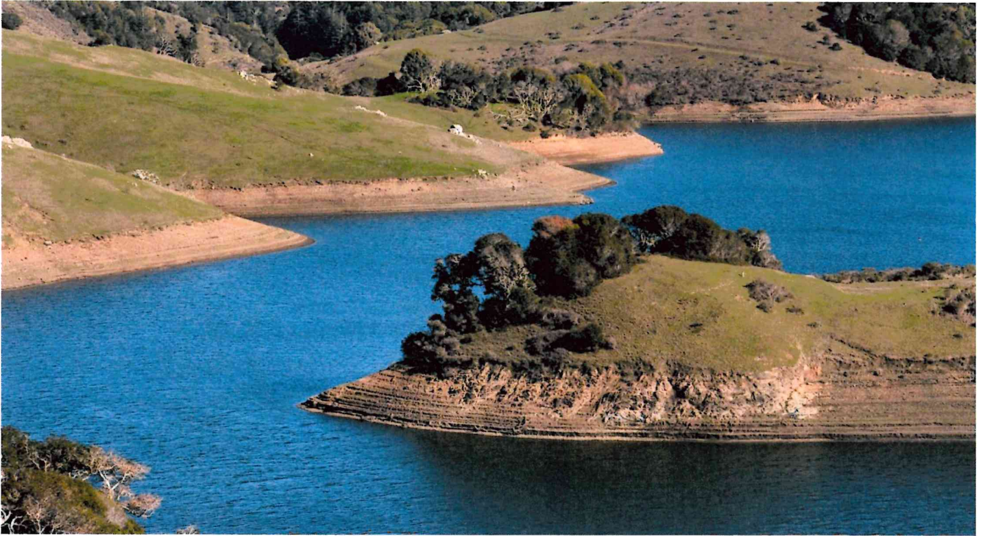
The Soulajule Reservoir in northwest Marin County. One supply option looks at pumping water from Russian River to Soulajule Reservoir. SHERRY LAVARS — MARIN INDEPENDENT JOURNAL, FILE
