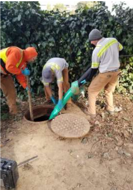
RVSD staff removing plug
