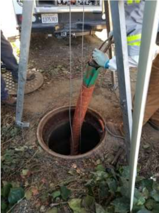
Inserting the 8' Fiberglass Repair
