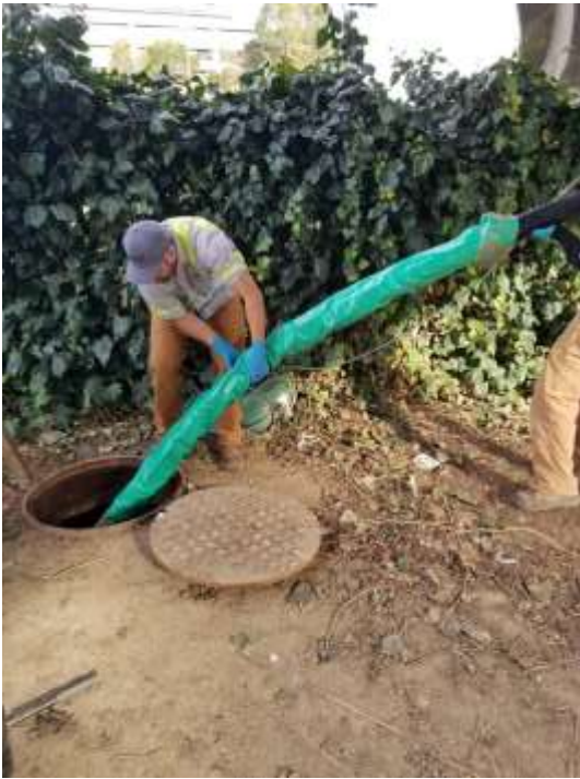
RVSD staff removing plug
