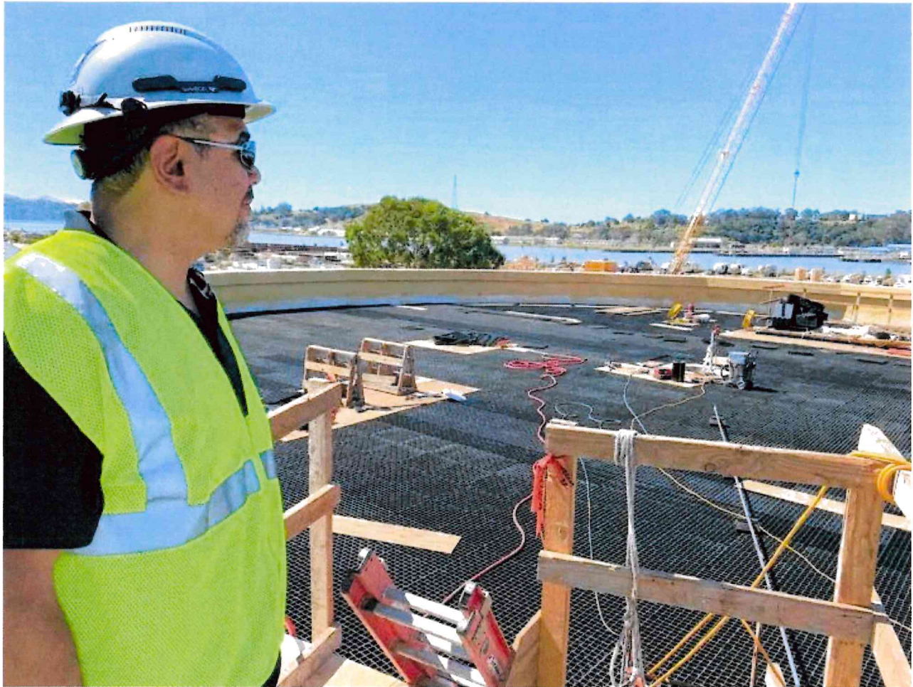
Orlando Cortez, operations superintendent at the Vallejo Flood and Wastewater District, looks at a biotower that's being rehabilitated and creating odors in the city.
